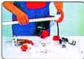
Step 3 remove both pipe and fittings when the welding time is over and insert pipe in the fitting
